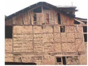
Fig. 2. Dhajji – Diwari in a typical Kashmiri House.
